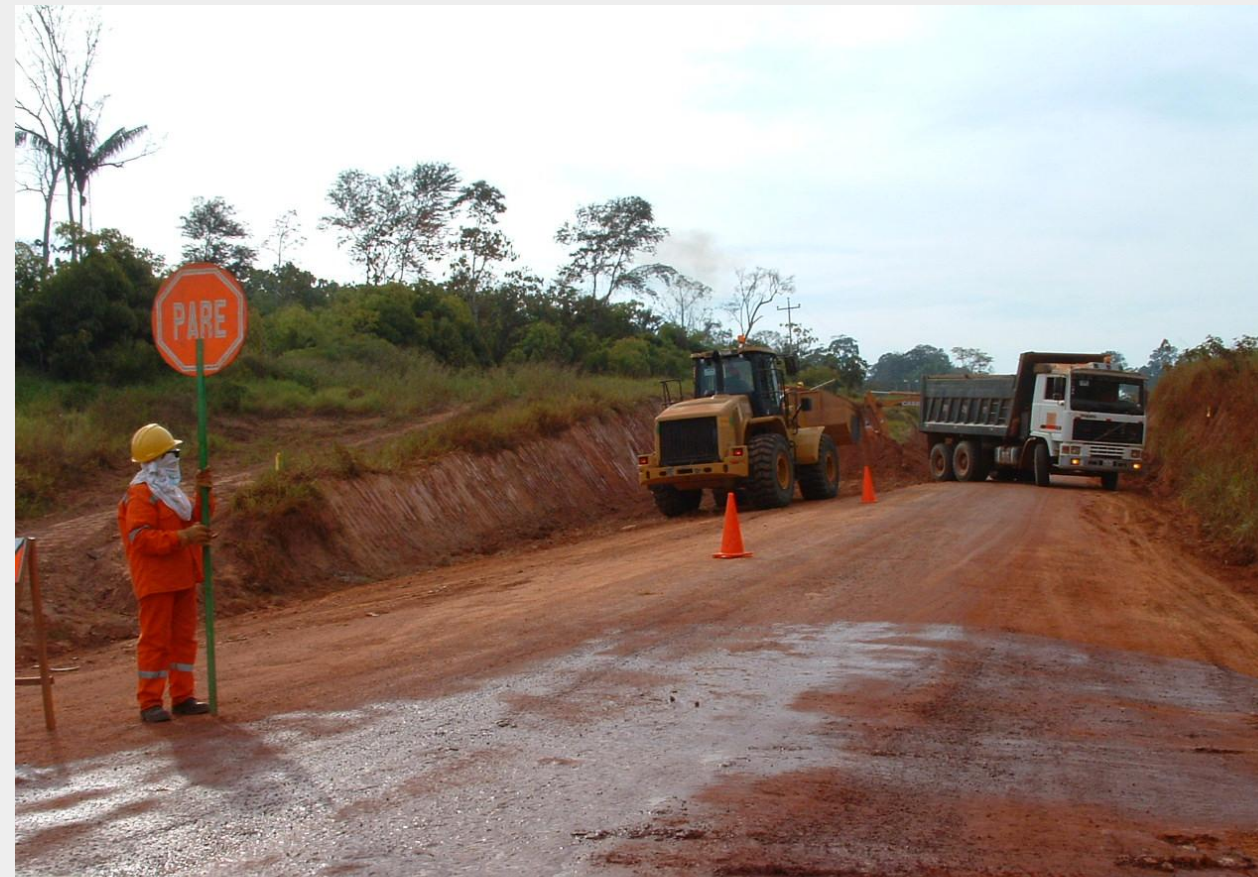
Fig. 2 (above): Road construction along the interoceanic highway (Salisbury, 2007).
